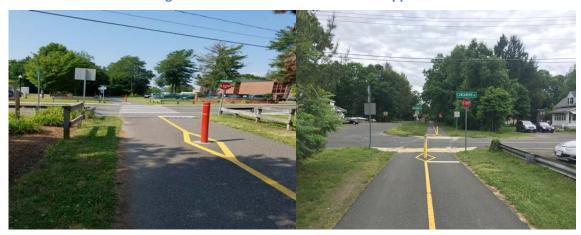
Figure 9: Bollards at Shared Use Path Approaches
