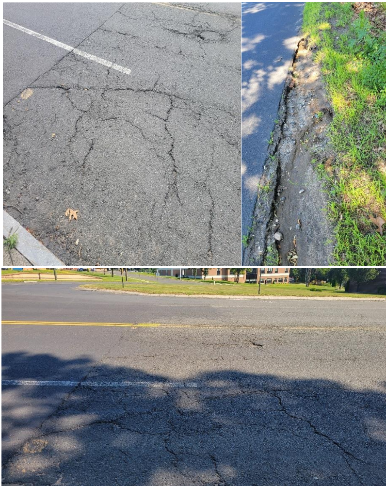
Figure 5: Mill Street Pavement and Pavement Markings
