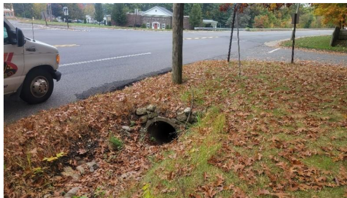
Figure 6: Culvert in the Southwest corner of the Intersection
