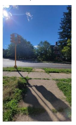
3. A single vehicle crash was reported when a motor vehicle crashed into the utility / signal pole on the northeast corner of the intersection between the Dartmouth Street and St. James Avenue. The granite curbing along this corner of the intersection was noted to have very little reveal. New curbing in this area would preserve the edge of pavement and better define the intersection.
